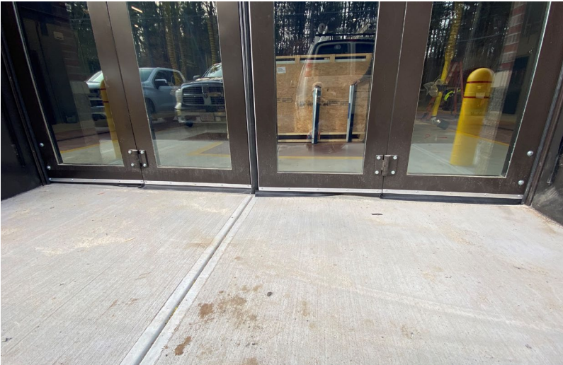
Bifold door bottom seal installation
