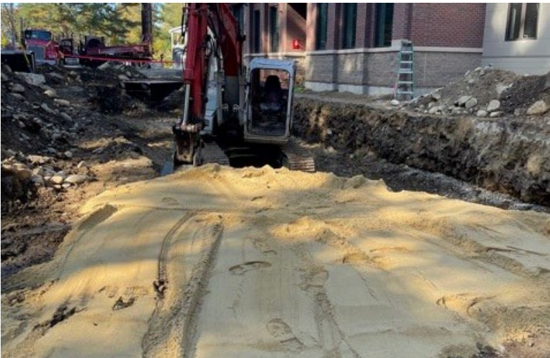
More septic system installation
