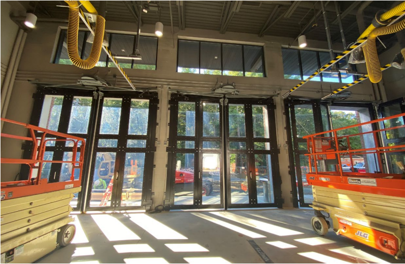
Bifold door installation
