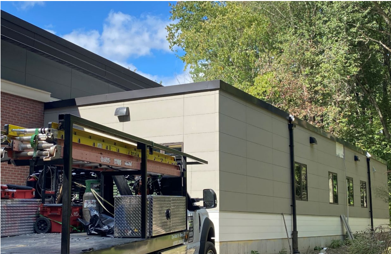
Metal roof edge flashing installation
