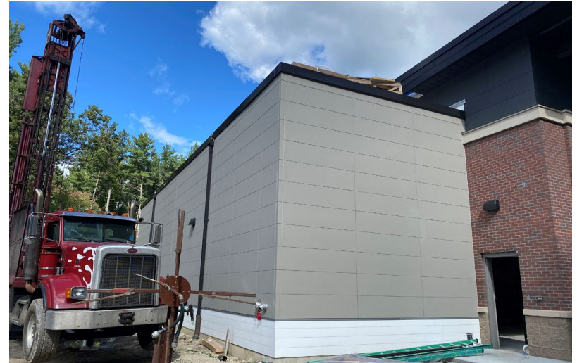
The other side metal roof edge flashing installation
