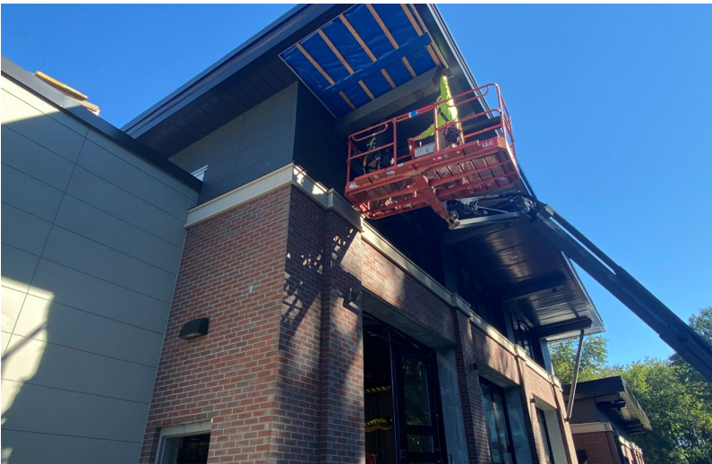
Nichiha siding and soffit installation
