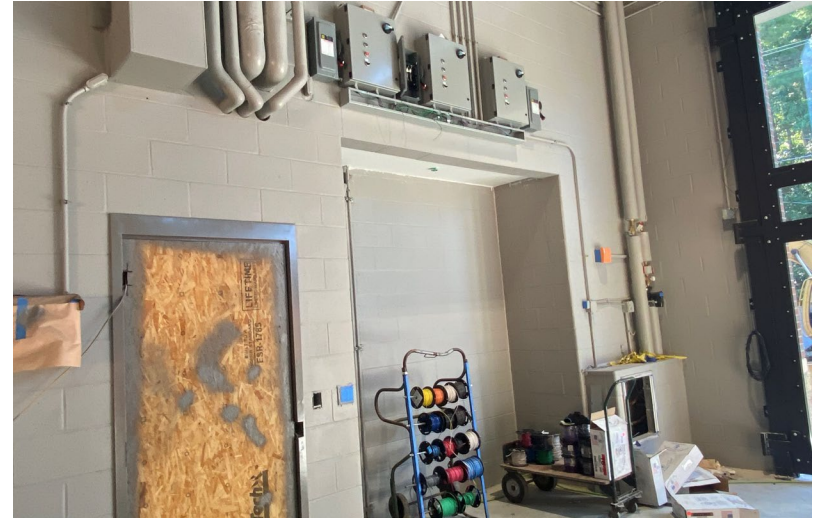
Door controls installation
