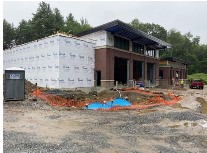
Overview of building from southwest
