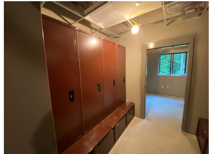
Duty lockers installed. Bench and top to be installed
