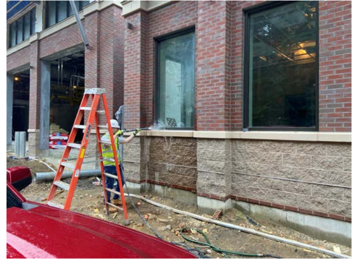
Water testing at watch room
