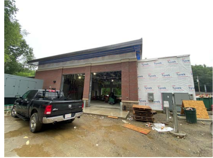
Overview of northwest side of building
