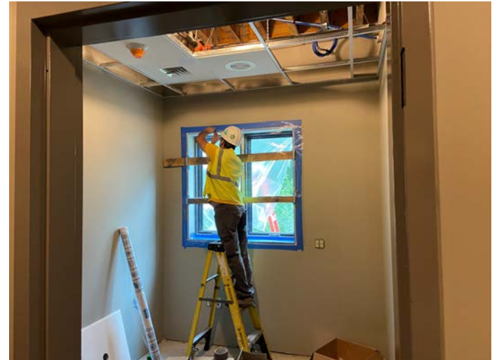
Set up for bunk room window testing
