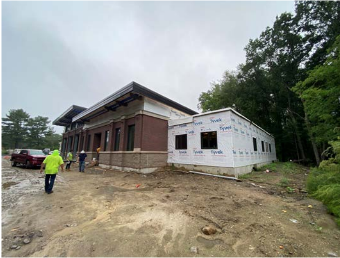
Overview of building from southeast
