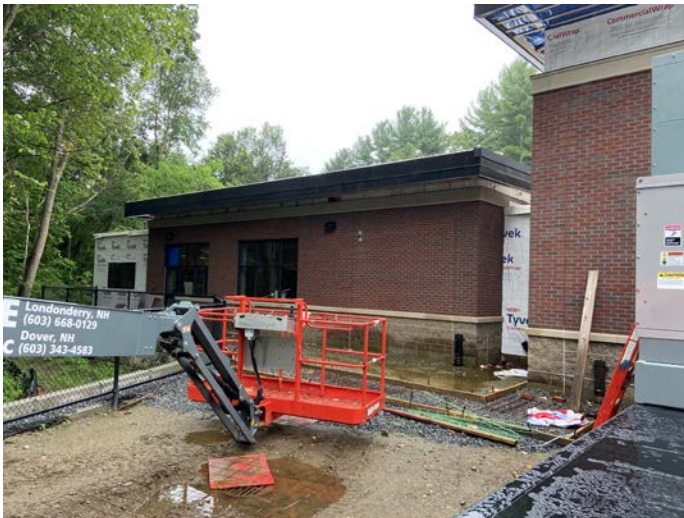
Overview of northeast side of building
