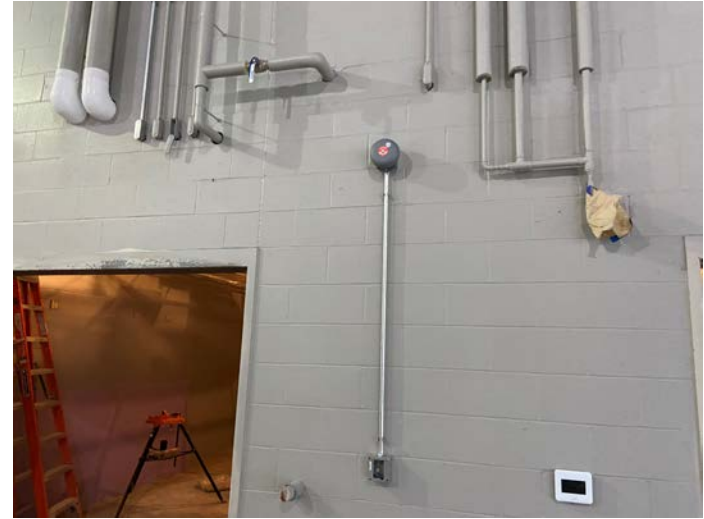
Fire alarm bell installed
