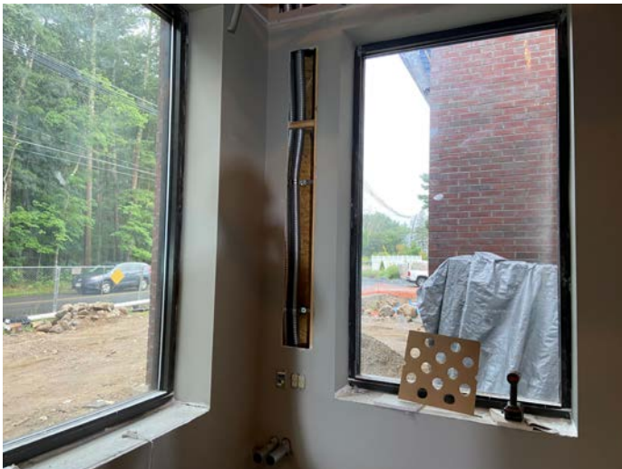
Fire alarm conduits installed
