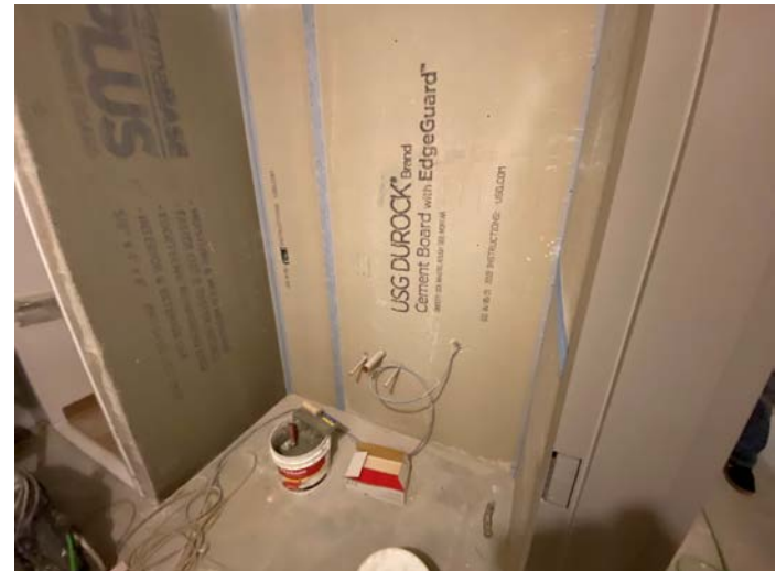
Taping bathroom wall joints for thin set mortar
