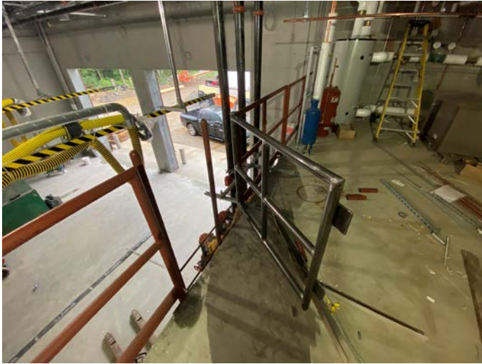
Mechanical mezzanine swing gate fabricated
