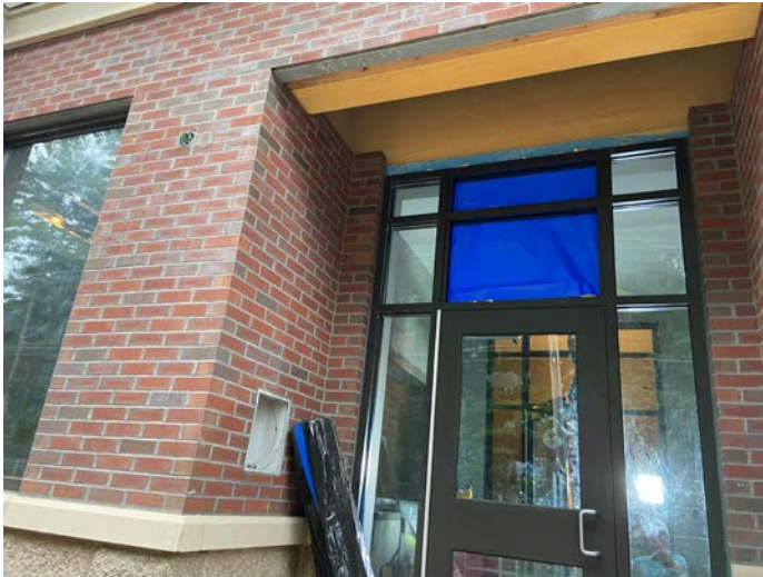
Temporary enclosure for interior climate control
