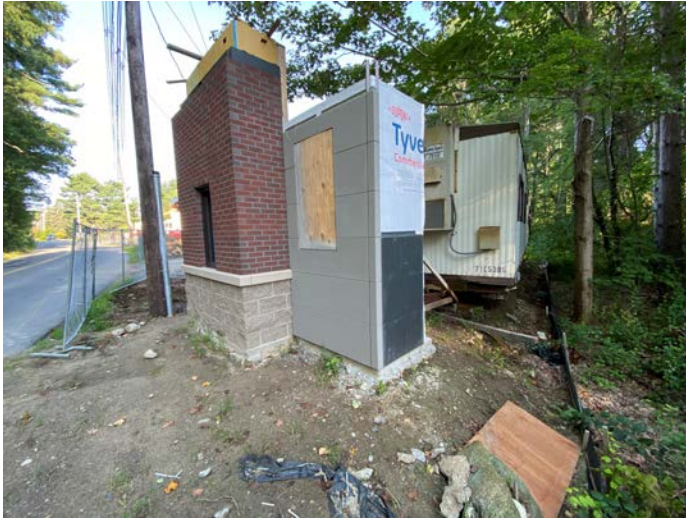
Installation of Nichiha panels on mockup
