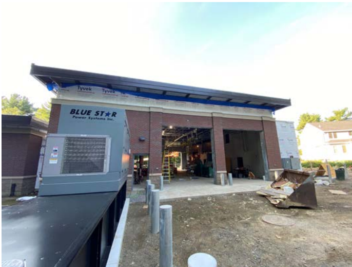
Overview of north side of building
