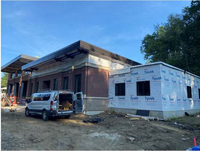
Overview of building from southeast
