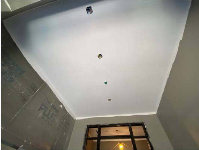
Vestibule ceiling primed
