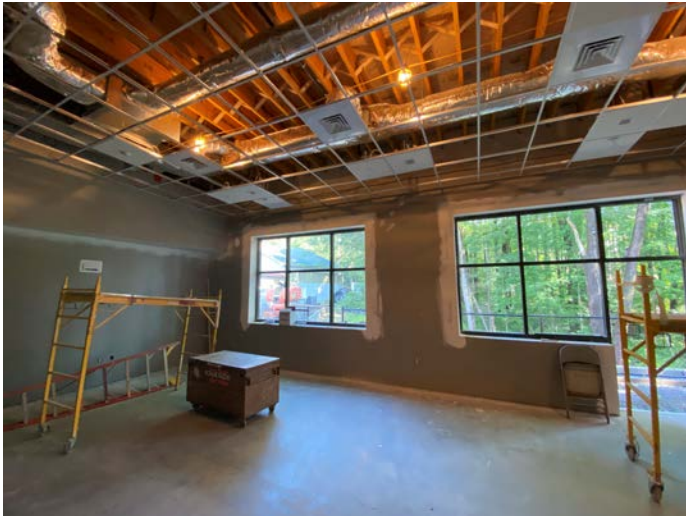
Overview of day room
