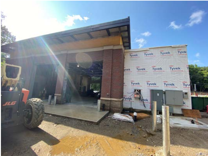
Overview of northwest side of building
