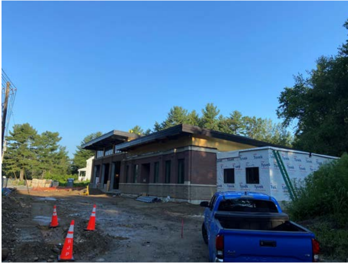
Overview of building from southeast
