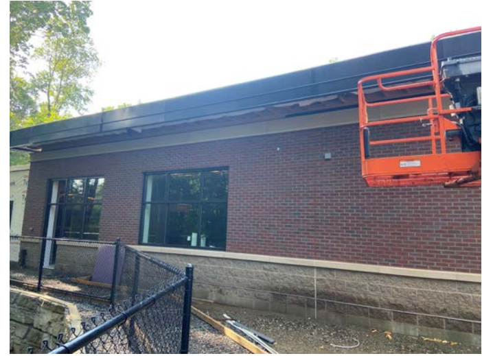
Overview of northwest side of building
