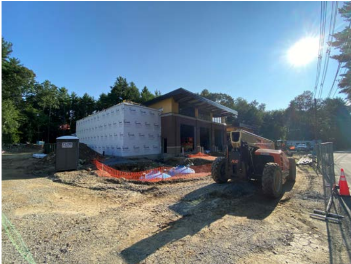
Overview of building from southwest
