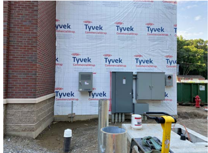
Installation of exterior electrical cabinets
