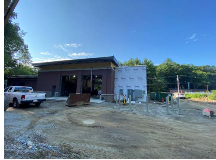
Overview of building from north
