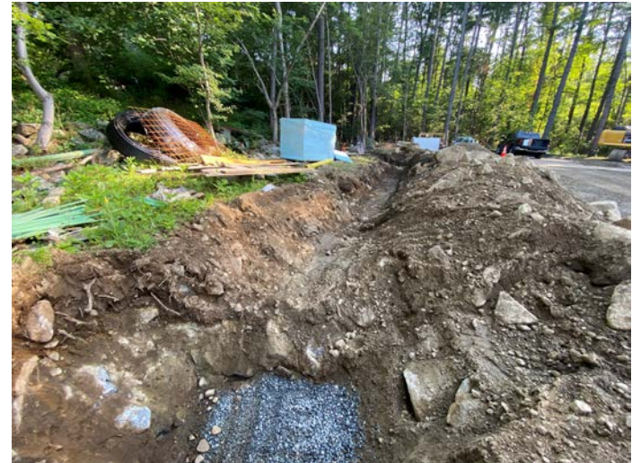
Excavation for north parking lot site lighting and conduits
