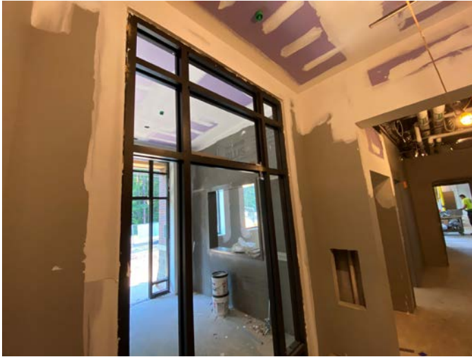
Drywall and frames installed at vestibule
