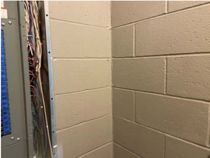
Typical interior sealant installed
