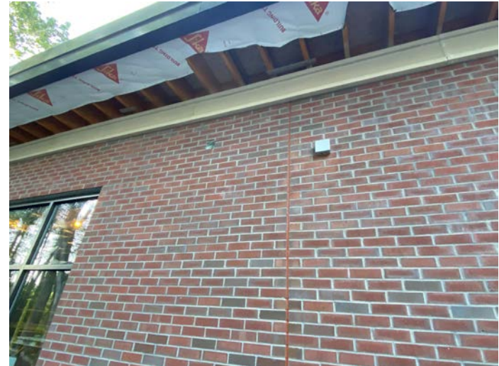
Typical exterior sealant installed
