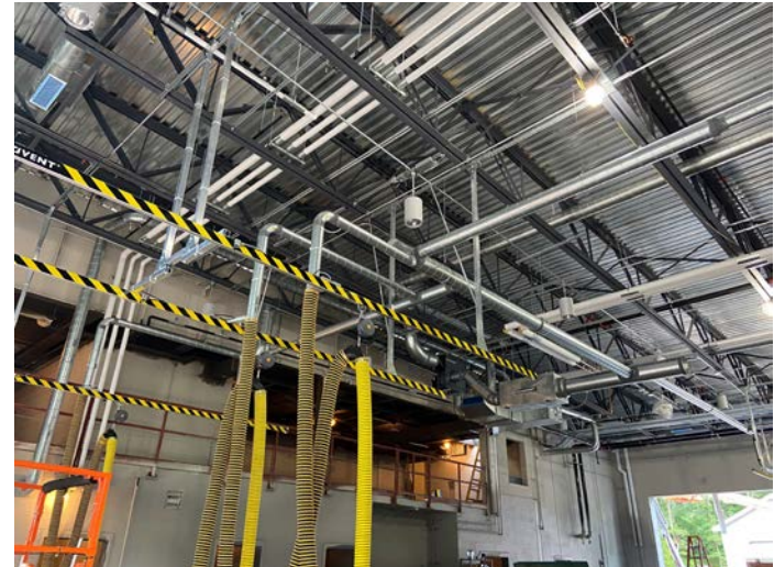
Vehicle exhaust system installation
