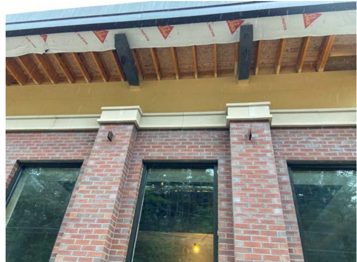
FRP Cornice on south side of building
