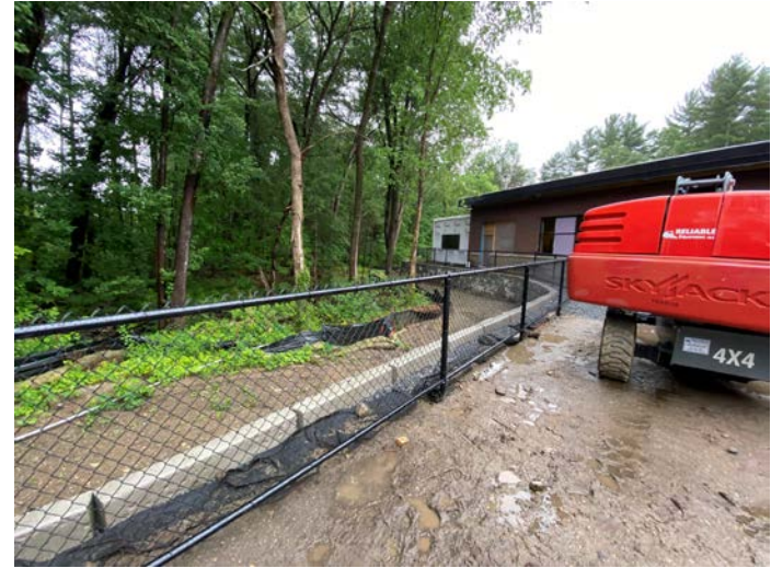
Fence along retaining wall
