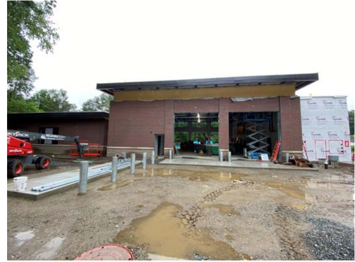
Overview of building from north
