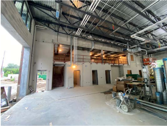
Block filler painting on west side of apparatus bay
