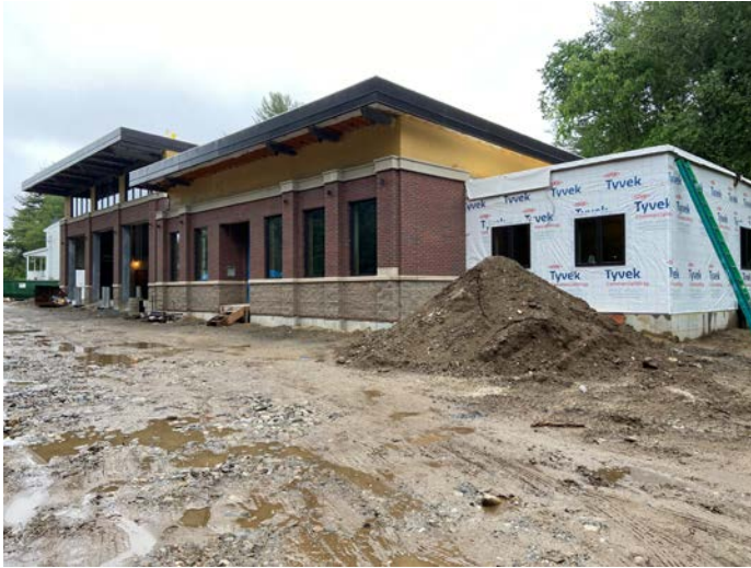
Overview of building from southeast
