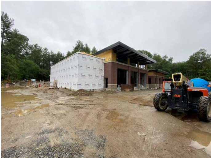
Overview of building from southwest
