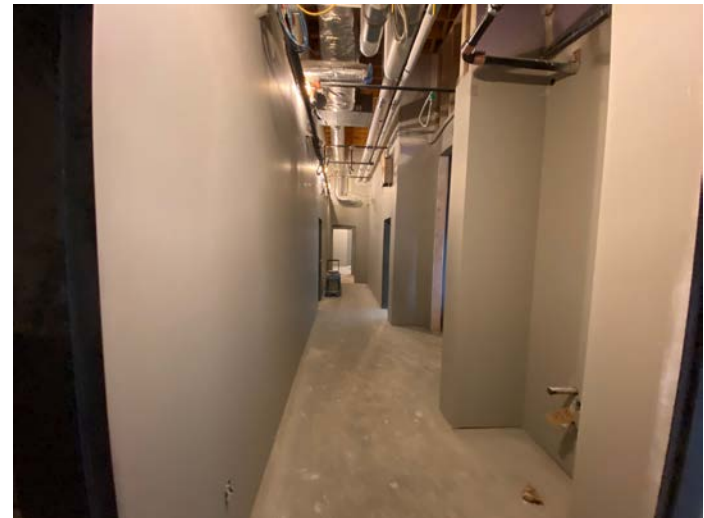
Hallway between watch room and study
