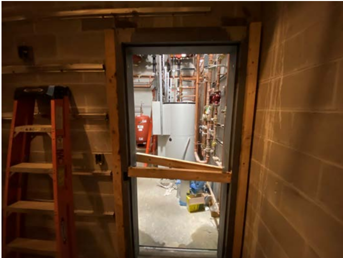
Grouted door frame at mechanical room
