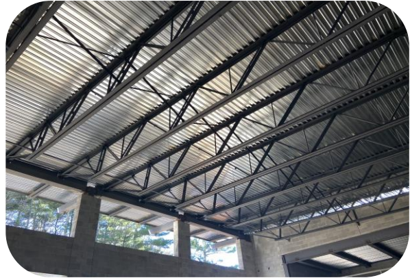
Steel roof joists in apparatus bay looking southwest
