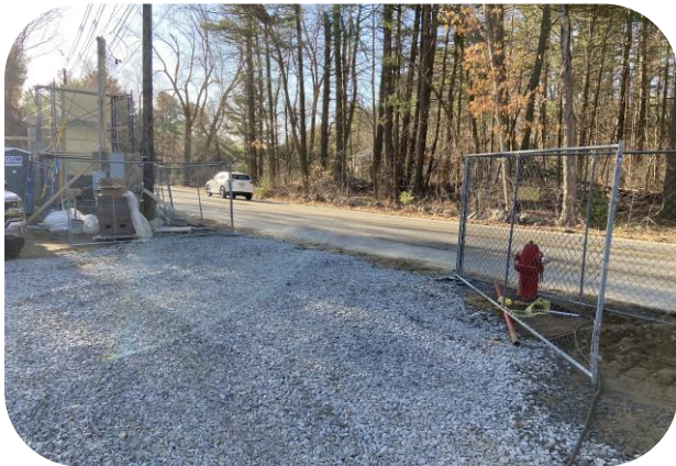
Fencing and crushed stone at southeast construction entrance
