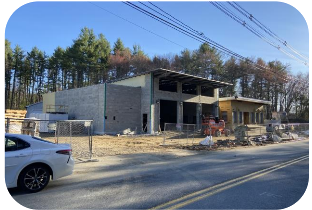
Overview of building from southwest side of site
