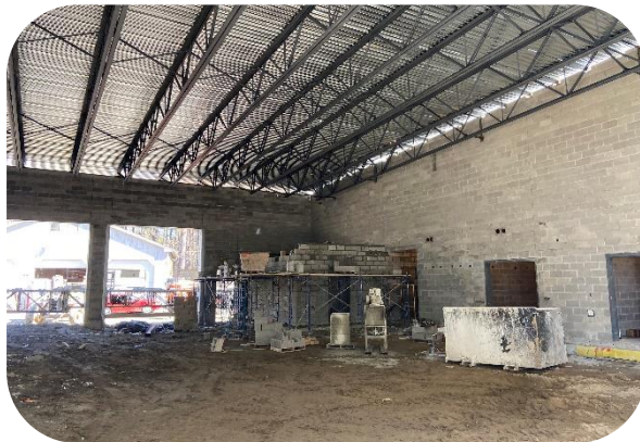
Masonry construction in dirty laundry room
