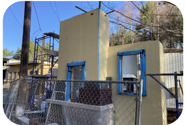
AVB and masonry facade installation at mock-up
