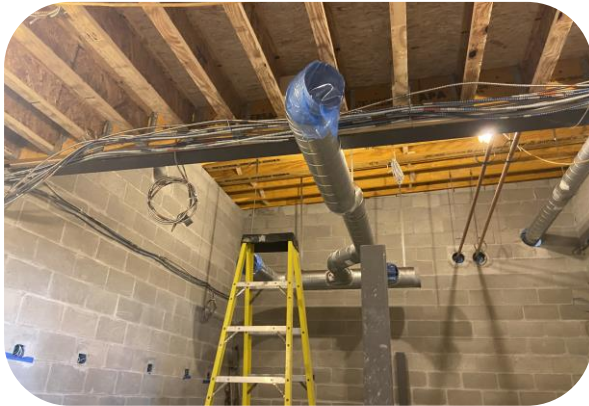
MEP rough-ins in gear room
