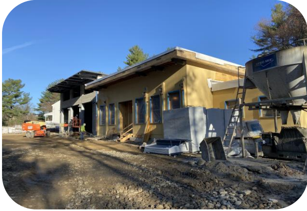
Overview of east side
