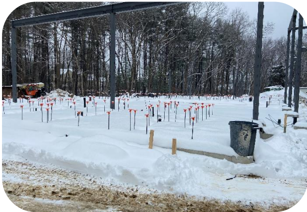
Overview of building from west side
