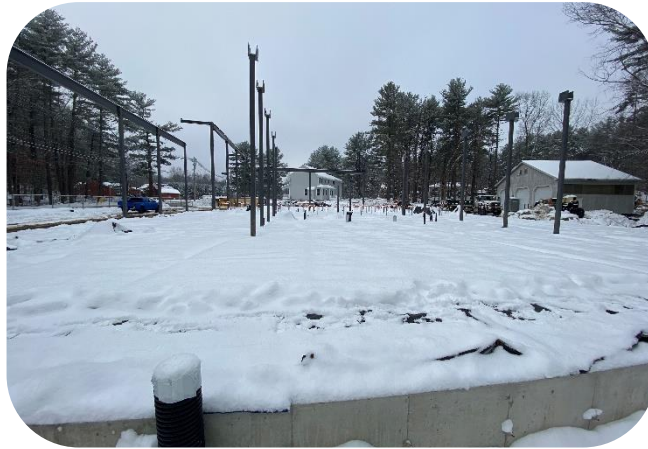
Overview of building from east side
