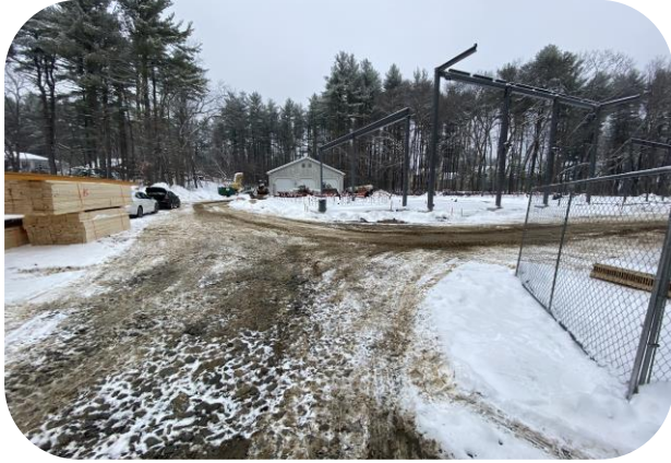
Overview of site from southwest corner
