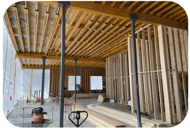
Interior wood framing and LVL corrective action
