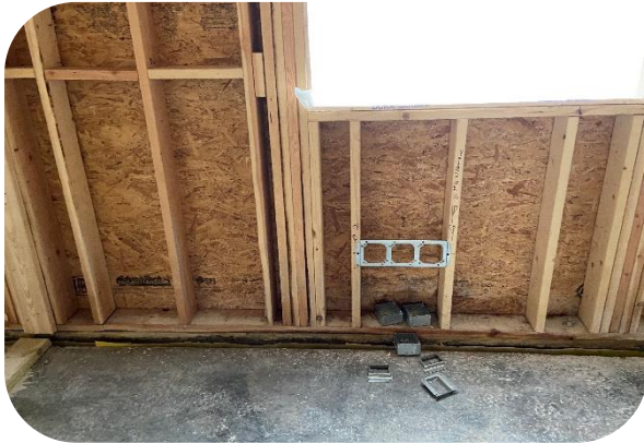
Electrical rough work on east side of building
