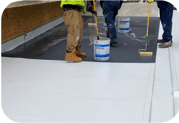
Installation of waterproofing in low roof area
