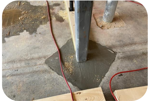
Concrete placed in column box
