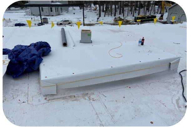
Waterproofing and mechanical curb installed on living area
