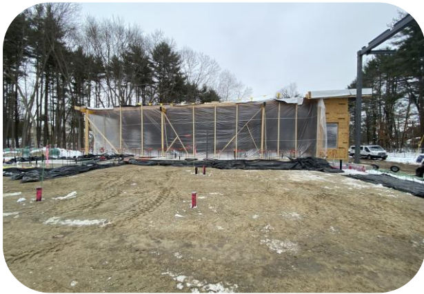
Overview of building from west side
