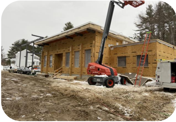
Overview of wood construction from southeast
