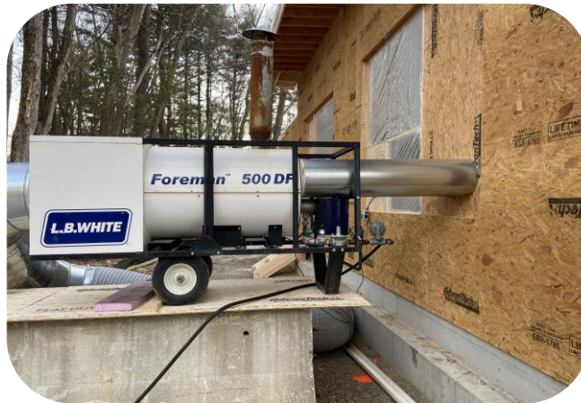
Heater set up on north side of building
