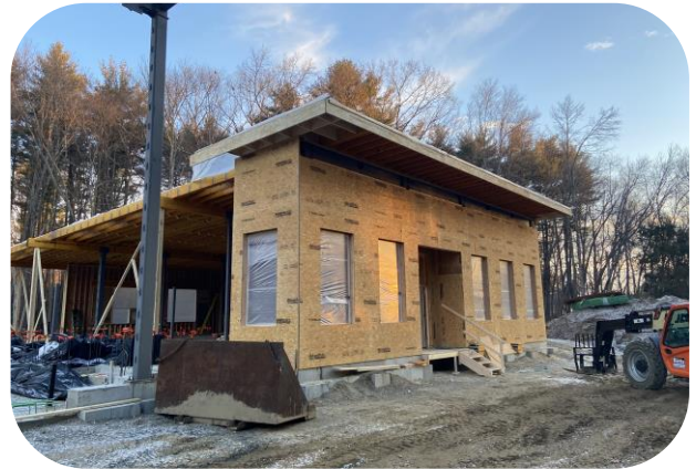
Overview of wood construction from southwest
