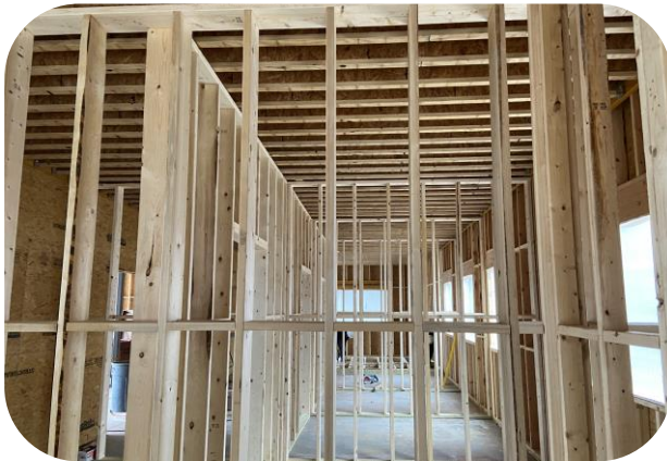
Interior framing in low roof area
