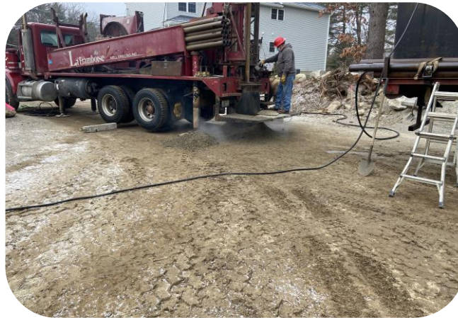
Geothermal well drilling
