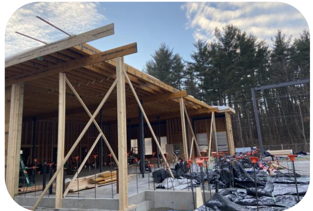
LVL joists installed on east side of building
