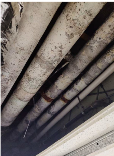
Mold growth on piping in ceilings
